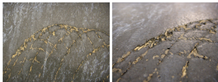
Figure 2 – Examples of high pressure cleaning wand damage to roll covers
