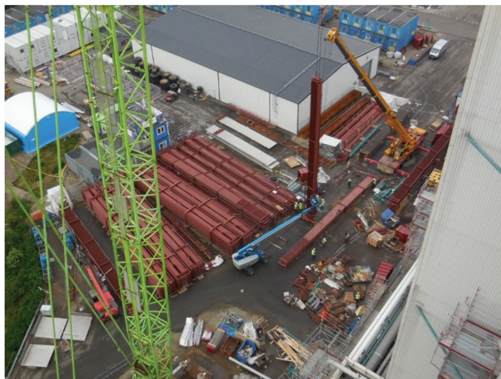
Figure 13. New heating surfaces waiting to be hoisted into the recovery boiler
