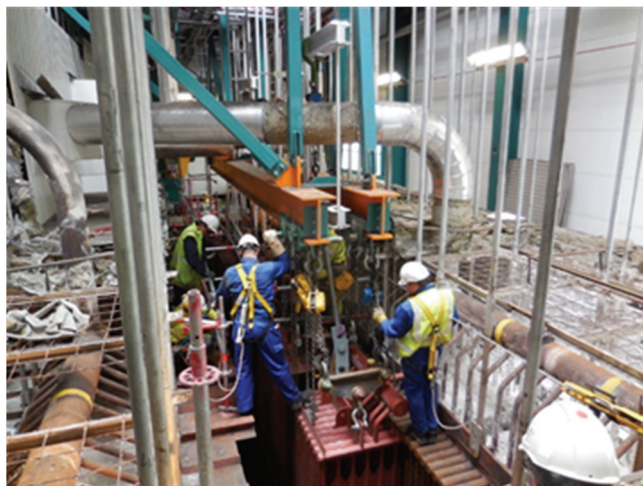
Figure 15. Despite challenges during the outage, the focus on safety was high.
