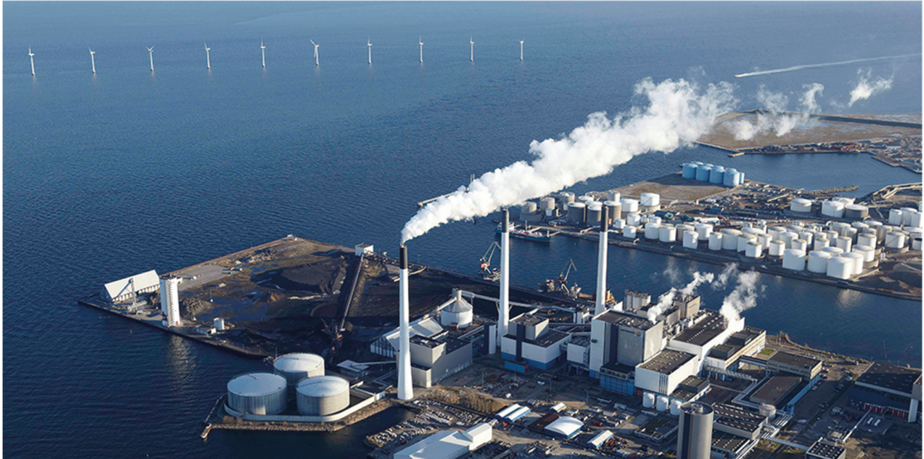
Figure 3. Amagerøerke located at the tip of the island of Amager, Copenhagen
