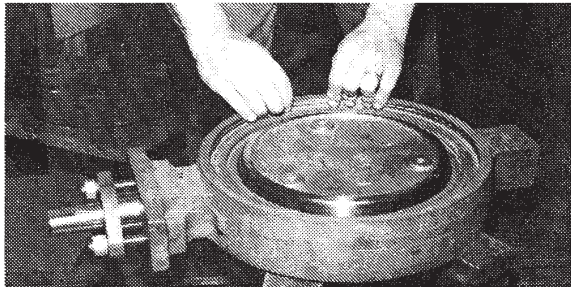
Placing Spring Into Groove
