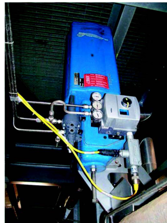
B1-series actuator with ND controller at a customer site
