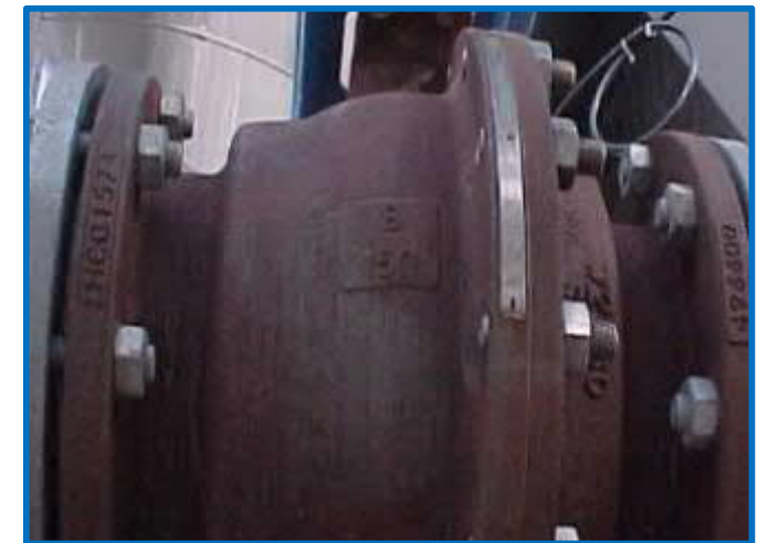
Improper weld repair
