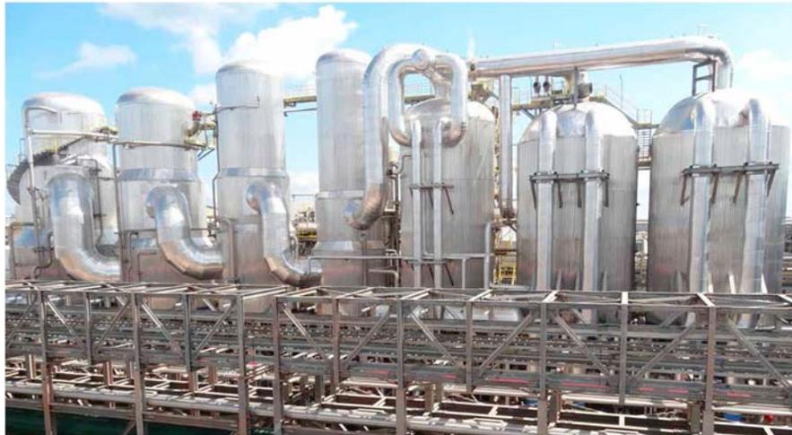
**Figure 3.** TUBEL technology at the Suzano Papel e Celulose evaporation line
