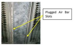
Figure 14. Plugged air bar slots (pre-rebuild)
