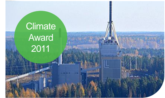
World's largest Waste-to-Energy Gasification Plant, Lahti Energia
