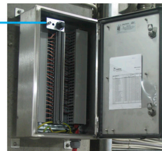
Connection to remote monitoring switch box
