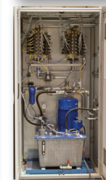
Figure 11. Using a smaller HPU and an accumulator reduces equipment and field piping costs.
