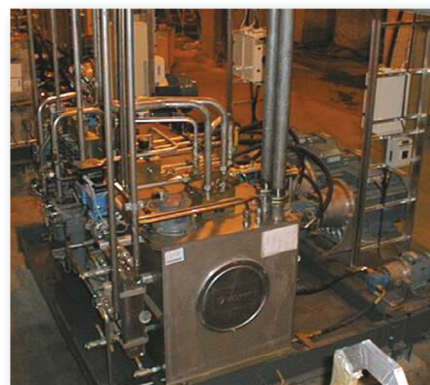
A typical large loading unit in an analog hydraulic system is located in the basement.
