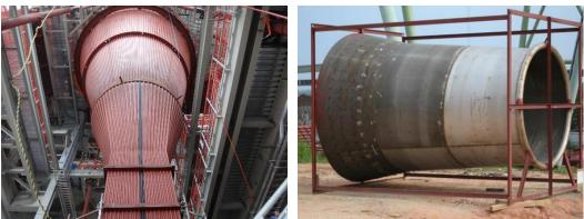
Figure 9. Left: water-cooled membrane cyclone before installation of insulation. Right: cyclone vortex finder before installation.
