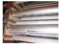
Figure 14. Finishing superheater with double tube design
